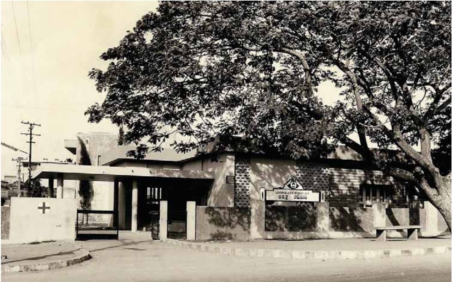
1970: The dispensary building at Adegodi, Bangalore, was the first-of-its-kind in the city built in a record time of four months by Mico for the benefit of local people.
